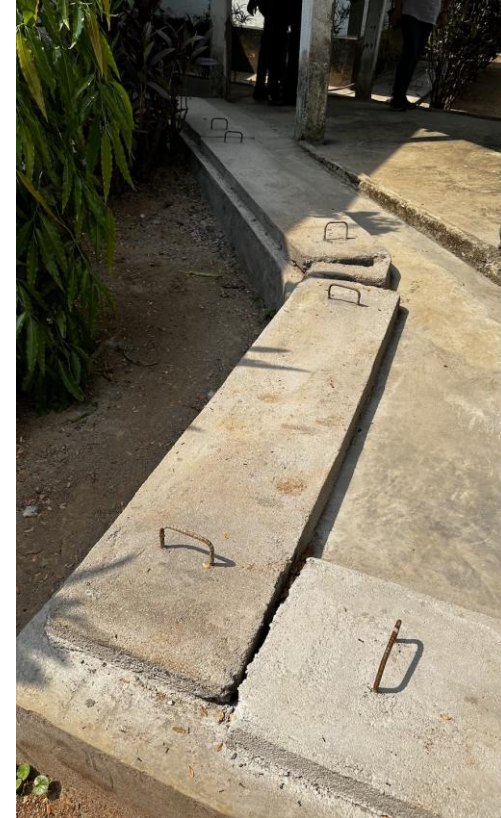
Slabs covering for drains
